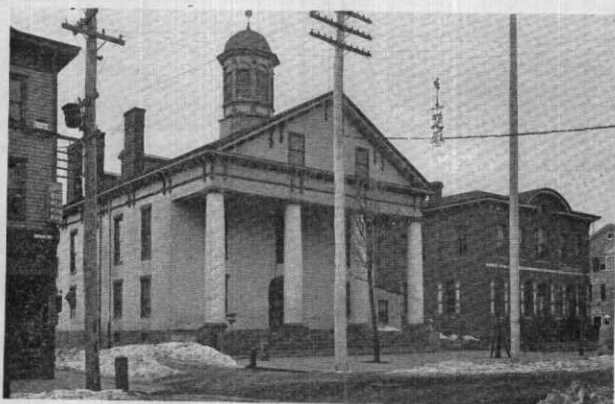
HUNTERDON COUNTY COURT HOUSE, FLEMINGTON.
